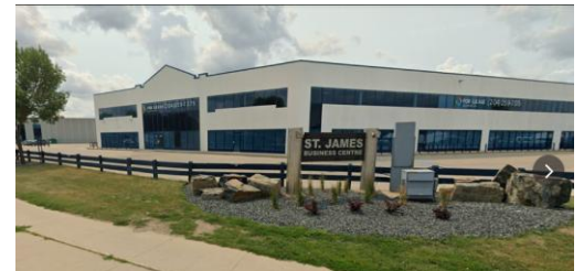
MANITOBA POSSIBLE building Free and Accessible Parking
